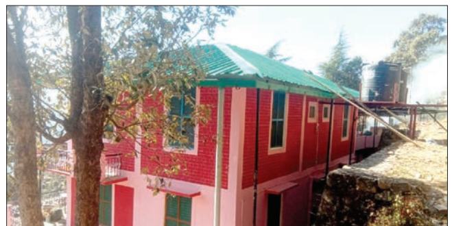
Renovated Convent at Damdeval
